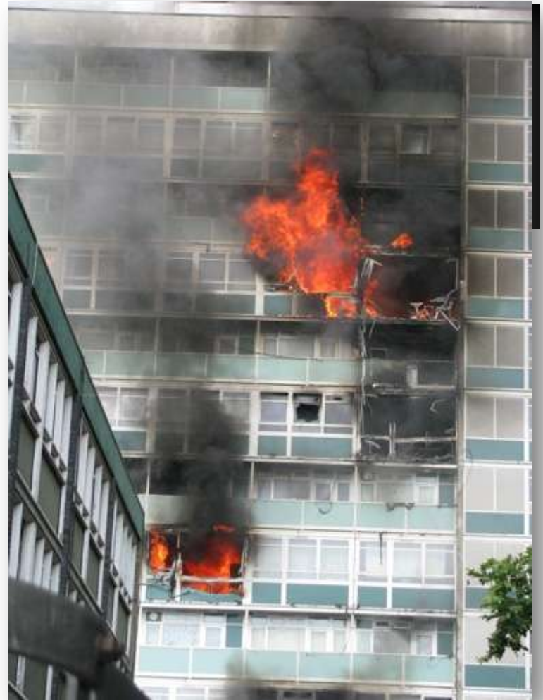
July 3 rd : Lakanal House Camberwell Source London :Standard
